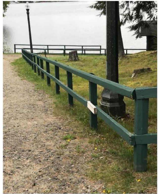
Existing handrail near toboggan shoot
