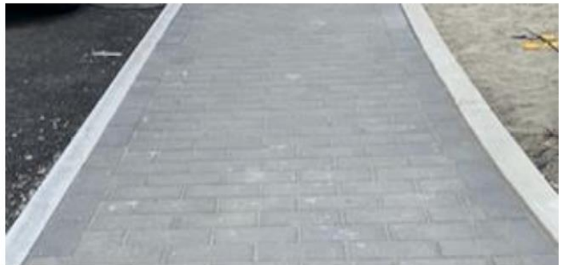
New gray pavers installed on Main Street in 2021
