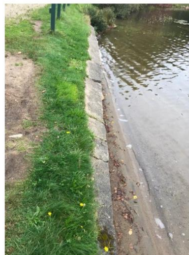
Existing northern retaining wall
