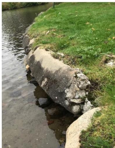
Existing southern retaining wall
